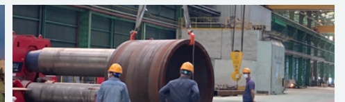
Joint Safety Inspection (Suncheon Plant)
